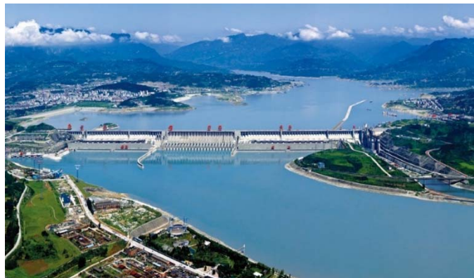
Fig 3. The Three Gorges Water Power Station on the Yangtze River in China, the presently largest on the Earth. The dam is 4 km long; the height difference is 126m.
