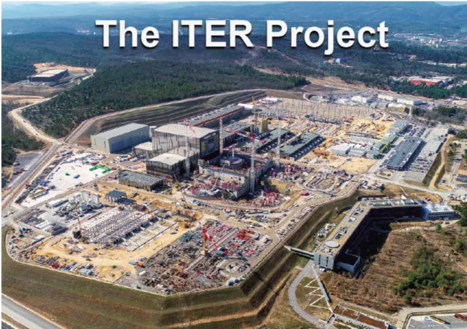
Fig. 8 The ITER magnetic confinement fusion project under construction in Cadarache, France
