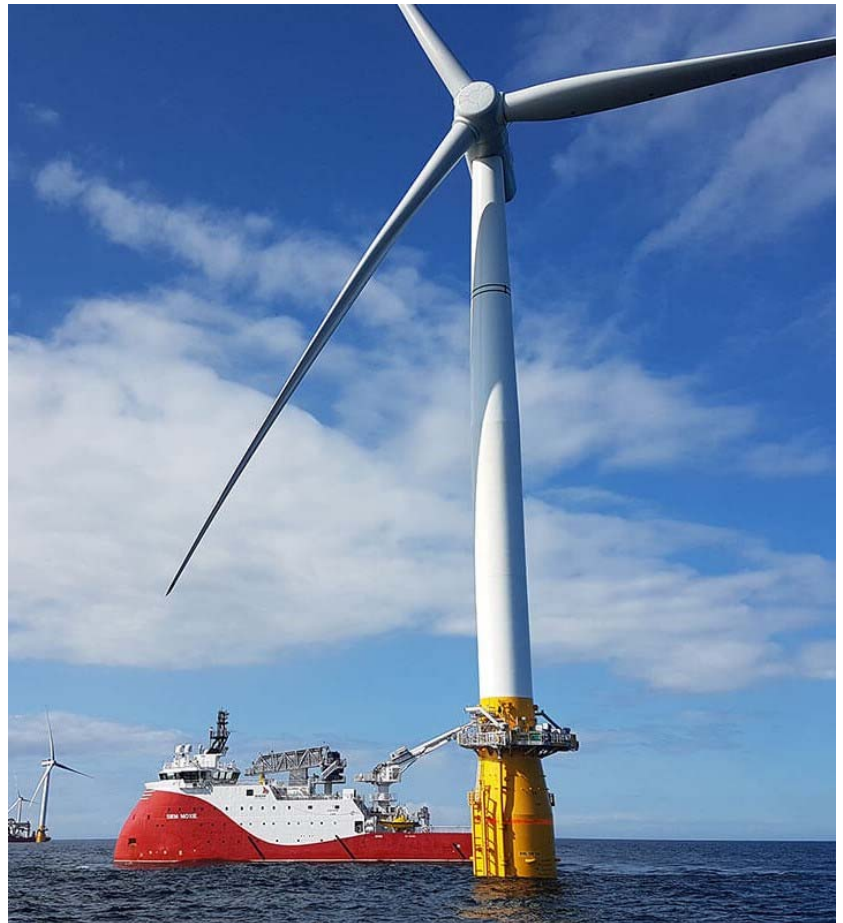
Fig. 6 An offshore wind-turbine of the HyWind floating pilotpark of Statoil, in front of Scotland.
